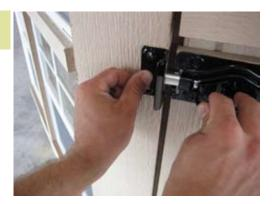
Install L-bracket to keep door closed. Use 1 1/4" blackhead screws to secure L-bracket.
