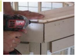
Insert 2 1/2" screws in an angle to tie top plates together.
