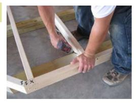
Once floor is square secure all the joist to the 4x4 runners as shown. Angle 2 1/2" screws thru joist into 4x4 runner. One on each side.
