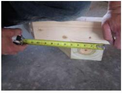
Hang tape over 4x4 and measure to corner of rim. Both reveels need to be the same.
