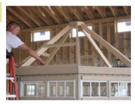
Secure bottom of rafters on top plate before doing the top.
