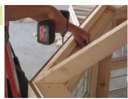
Secure 2x3 that is attached to rafters into 2x6 top plate with 2 1/2" screws.
