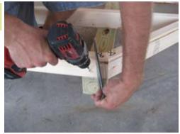
The 2 longest 4x4's need to be in the center. Keep 4x4 flush with rim and secure with 2 1/2" Zinc Screws as shown.
