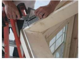
Secure rafter to top plate and make sure corners of rafters line up with the edge of the top plate as shown.
