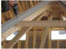
Secure with (3) 1 1/4" screws per side.
