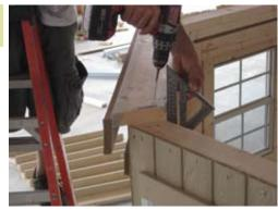
Install top plates as shown. Keep flush on the inside and make sure corners line up. Secure with 2 1/2" screws.
