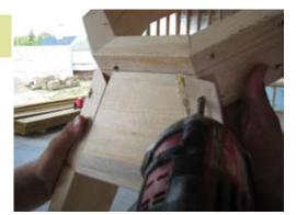
Install first rafter to Octagon as shown at pencil marked as shown.
