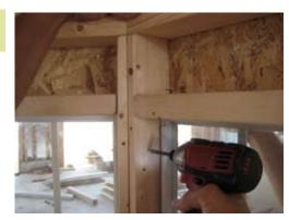
Make sure the inside corner is in place and secure with 2 1/2" Zinc screws as shown.
