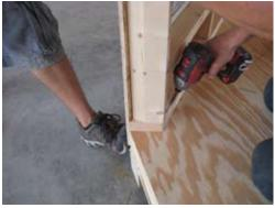
Secure wall panel A with 2 1/2" screws as shown. make sure corners line up and put pressure on the outside pushing in so wall is tight against floor as shown.
