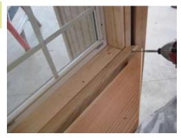
Next start installing shelves at corner as shown. Keep flush with top of window sill and secure with 2 1/2" screws. Deck screws are provided for treated shelves.
