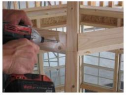
Halfway down from the top you will install 2x3's in between rafters as shown and secure with 2 1/2" screws.
