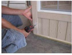
Secure all corners and bottom edge of siding with 1 1/4" screws 8" to 10" apart.
