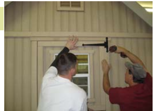
Next install top door first and make sure you have a 1/4" space on top as shown. Secure with 2 1/2" Black Headed Screws.
