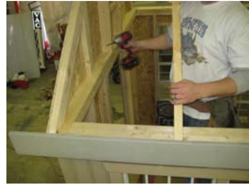
Next set Trusses.
