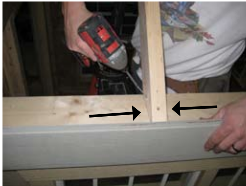
When securing truss use (3) 2 1/2" screws as shown (1) on top and (1) on each side of the truss.
