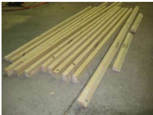
Next locate 2x3's for Purlins.
