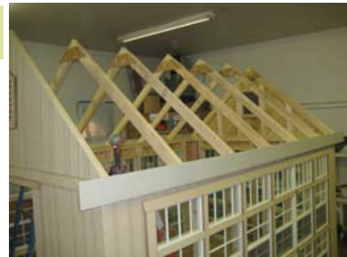
Trusses are completed.
