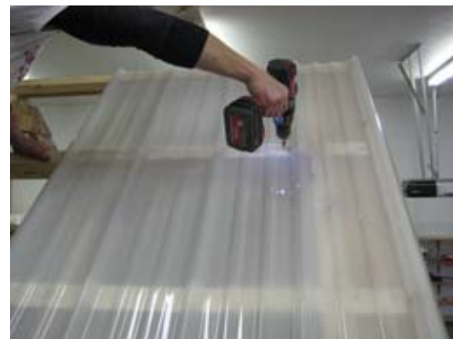
Secure with 1" screw on every purlin and beside every rib.
