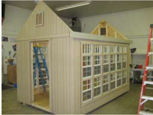
Gables are completed.
