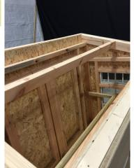
Pictured is the fastened roof purlin.
