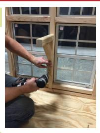
Fasten using 2 1/2" screws. And do the same for the second side center support beam. 20
