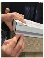
Be sure that the drip edge pieces align completely before fastening.
