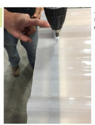
Attach using 1" white screws where holes are drilled in the roof.
