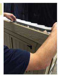
Attach the foam lining to the top of the roof sheeting at the front of the greenhouse, trimming away any excess foam.
