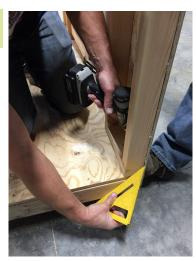
Make sure the front wall is square to the floor and fasten using 2 1/2" screws.
