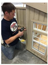
Fasten siding on corners and along bottom using 1 1/4" screws.
