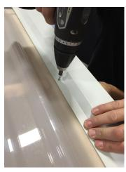
Attach the corner trim using 1" white screws 3 on top and 3 on the side.
