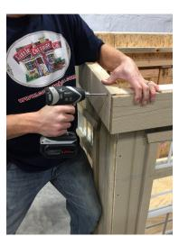
Fasten the sidewall to the back wall using 2 1/2" screws.
