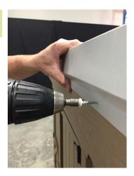
Do the same to fasten the front side using 1" screws.
