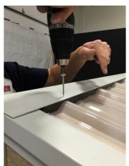
fasten the top side of the drip edge piece to the roof using 2" screws on all of the roof ridges and on each end.
