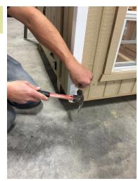
Attach the trim to the corners of the grennhouse using white aluminum nails.
