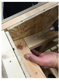
Fasten the sidewall to the front wall using 2 1/2" screws.
