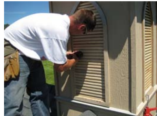
Insert 1 1/4" screws on each side.
