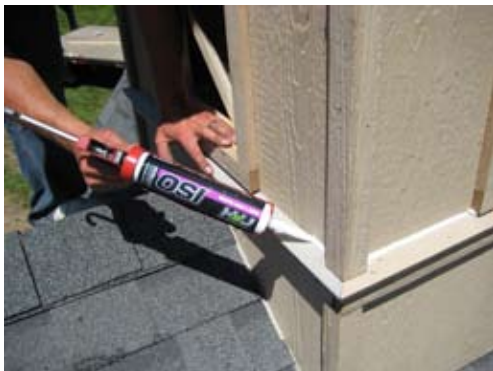
Run a bead of chaulking on all places where water can get to.
